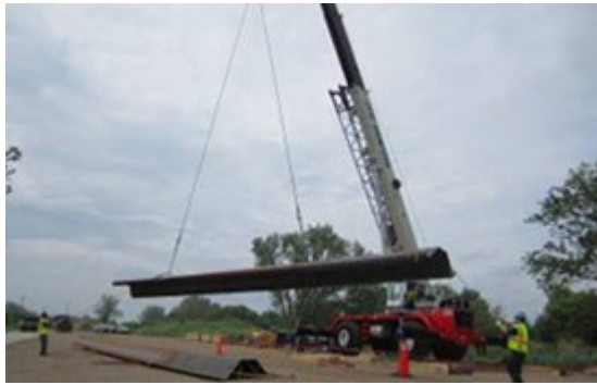
Steel panels are delivered to the lakeshore.
